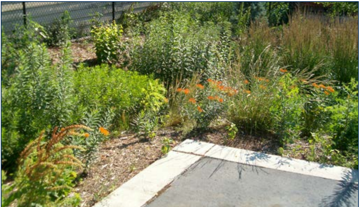
This rain garden receives, absorbs, and treats the runoff from the adjacent paving. (Brian Ash)
