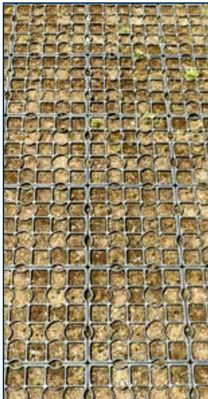
Three examples of pervious paving on driveways: concrete grid, plastic grid, and a "ribbon" driveway for treads only.
