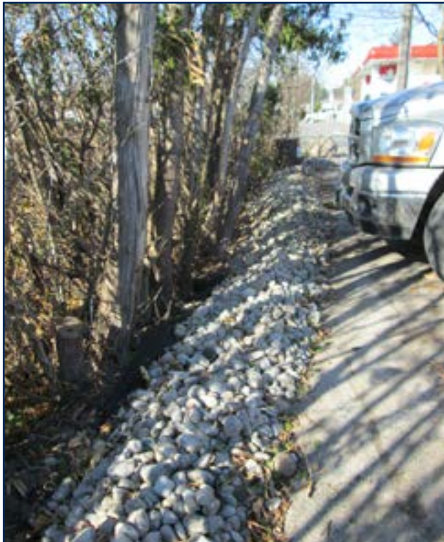
A soakaway trench beside a Port Perry driveway
