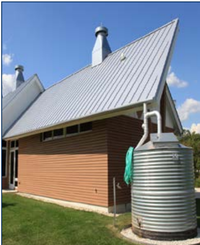
An example of a rainwater cistern. These are available in many shapes and sizes and may be above or below ground.
