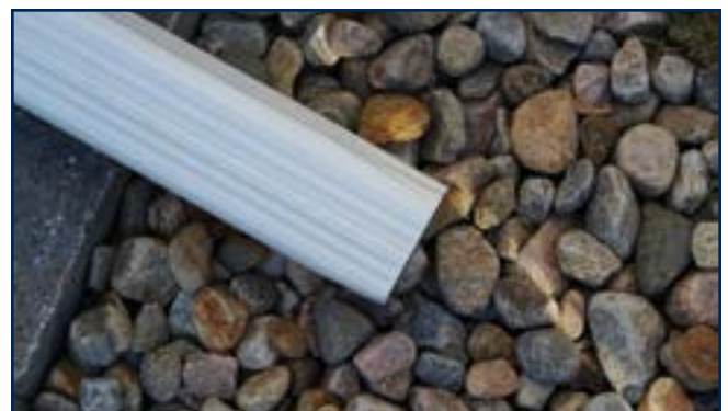
Direct downspouts to stone or vegetation.
