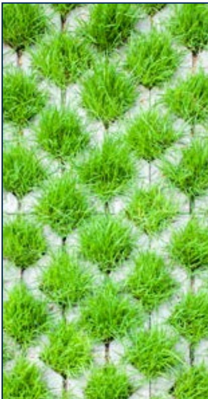
Three examples of pervious paving on driveways: concrete grid, plastic grid, and a "ribbon" driveway for treads only.
