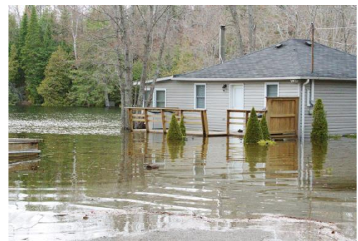
Flooding on the Gull River (Shadow Lake), 2013
