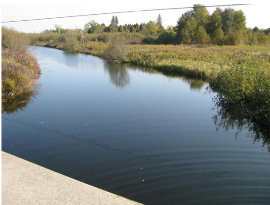
TLPR001 – looking d/s (October 2016)
