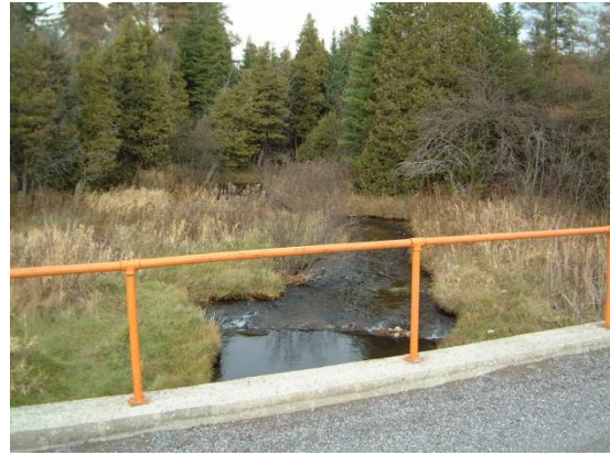
TLPRgauge – looking d/s (November 2001)
