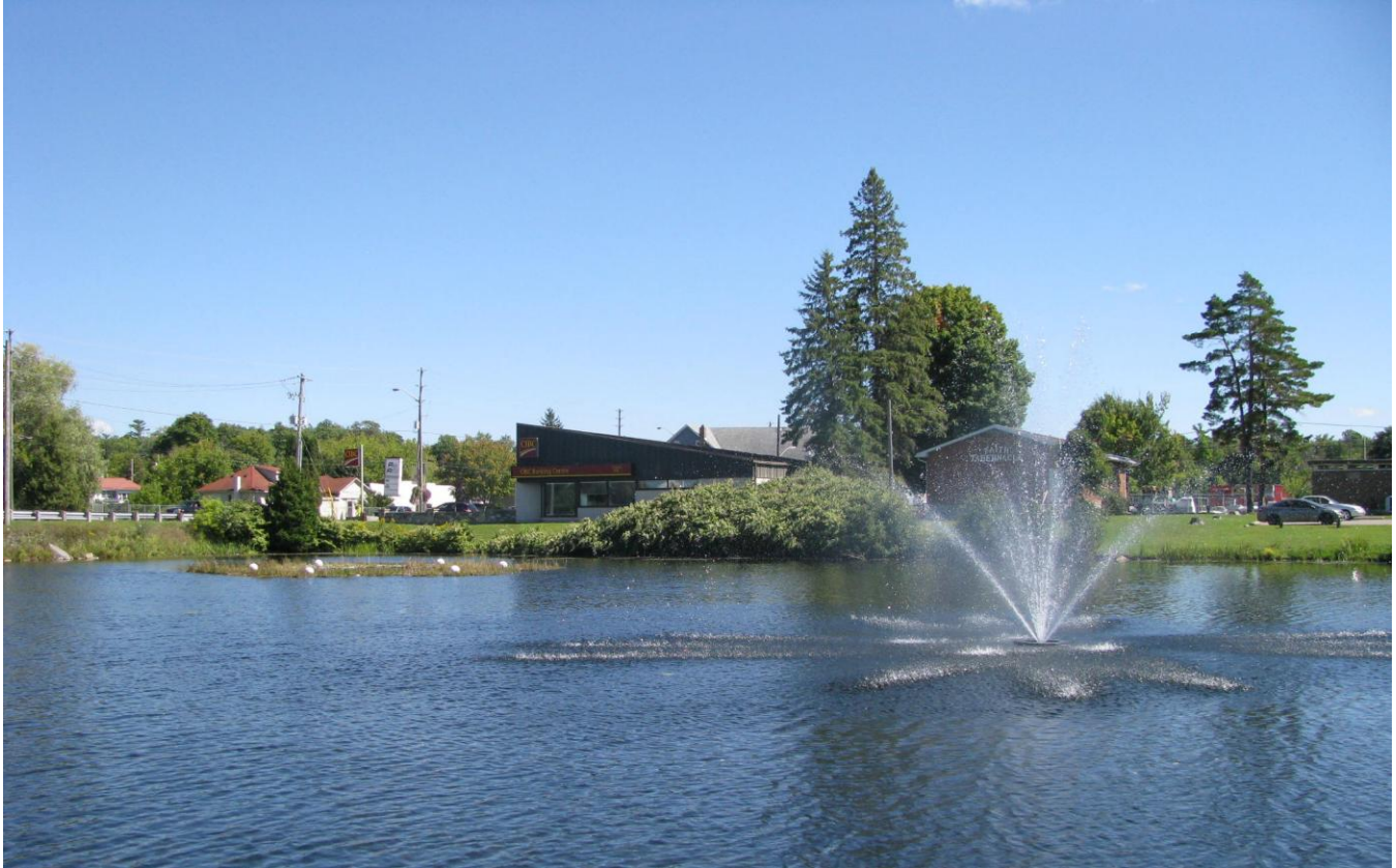
Showcasing innovative pilot projects to help improve water quality. Back left is a constructed wetland. Front right is an aeration fountain. (Outlet of Gull River, Coboconk, September 2014)
