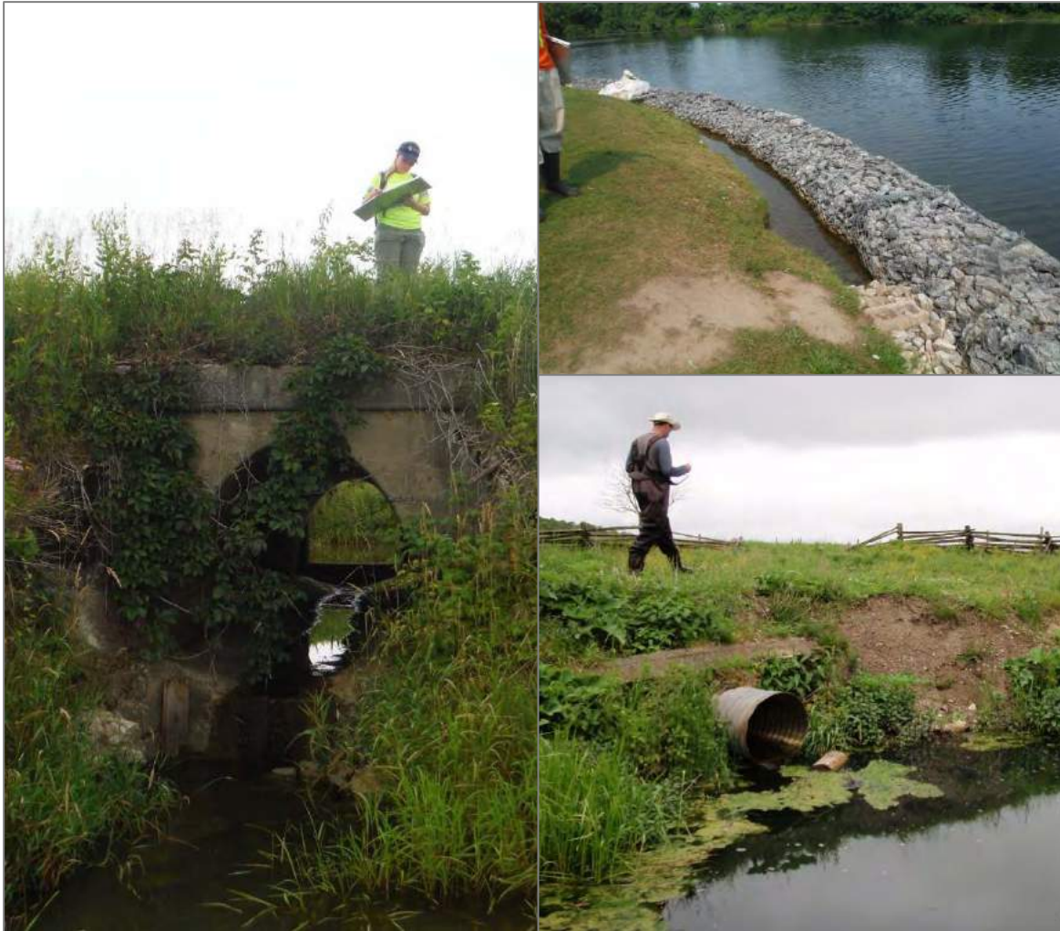
Figure 6-7: Examples of a weir, a failed bank hardening, and a perched culvert in the Whites Creek and Talbot River subwatersheds.
