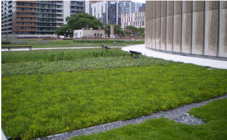
Figure 8 – An extensive green roof was installed on the podium level of the Toronto City Hall. Fully vegetated trays with 3" soil depths supporting low growing plants like sedums and 6" trays supporting grasses and flowering plants were used in the construction of the green roof. (Source: CVC)
