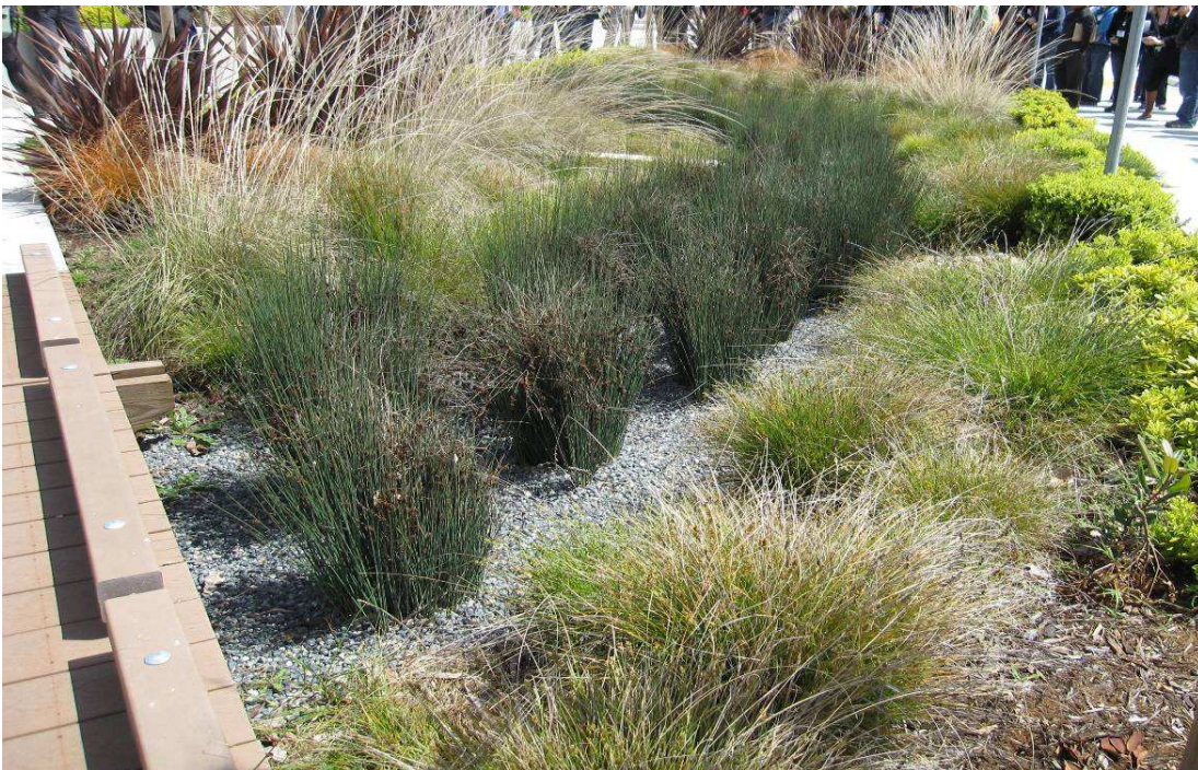
Figure 12 – Bioretention planted with ornamental grasses, Brisbane, CA. (Source: CVC)
