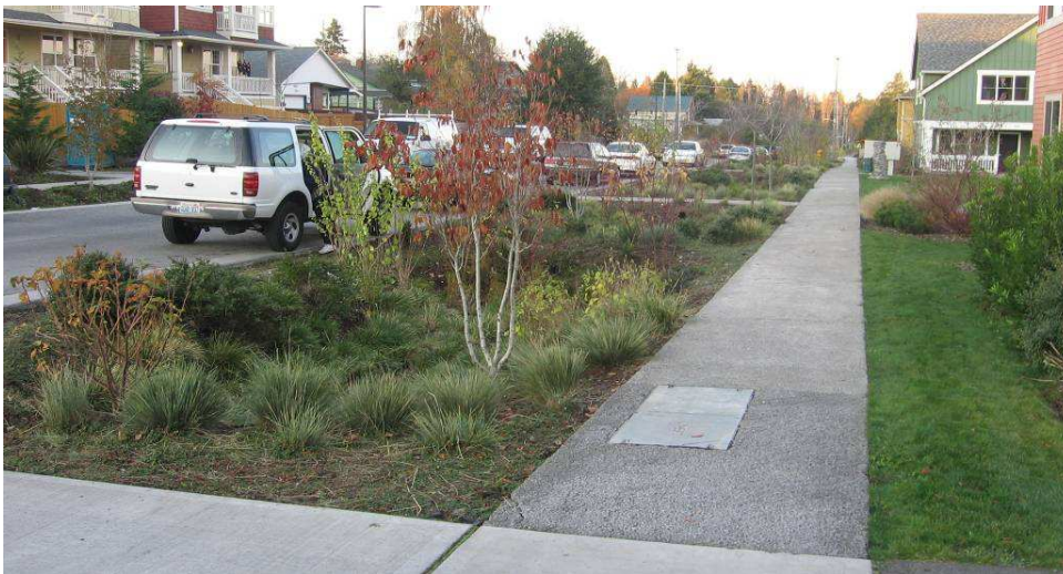
Figure 32 – Dry swale planted with a mix of herbaceous, shrub, and small trees in Seattle, WA (Source: CVC)
