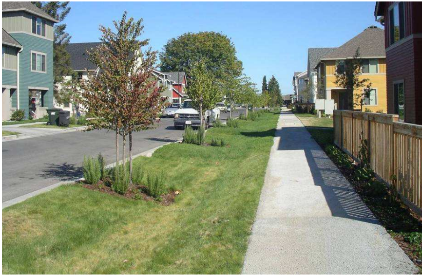
Figure 28 – Manicured shallow grass swale combined with areas of herbaceous plantings and trees between the curb and sidewalk in Seattle, WA (Source: SVR Design Company)
