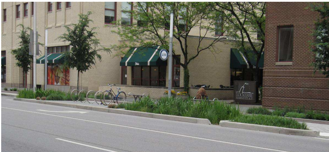
Figure 23 – Vegetated curb extensions collecting runoff from street in downtown Indianapolis, IN (Source: CVC)
