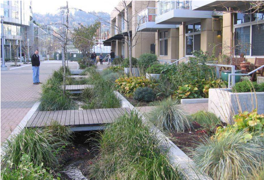
Figure 17 –Stormwater planter accepting runoff from high density urban development, Portland, OR (Source: CVC)
