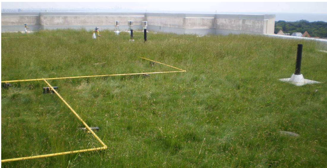
Figure 9 – An extensive green roof planted with grasses on the roof a condominium building in Mississauga, ON. (Source: CVC)
