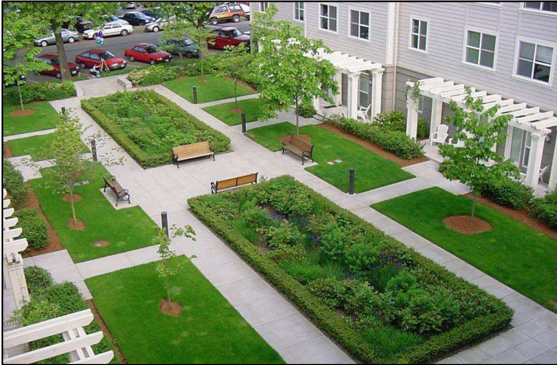
Figure 11 – Courtyard bioretention cells (Source: City of Portland Bureau of Environmental Services)
