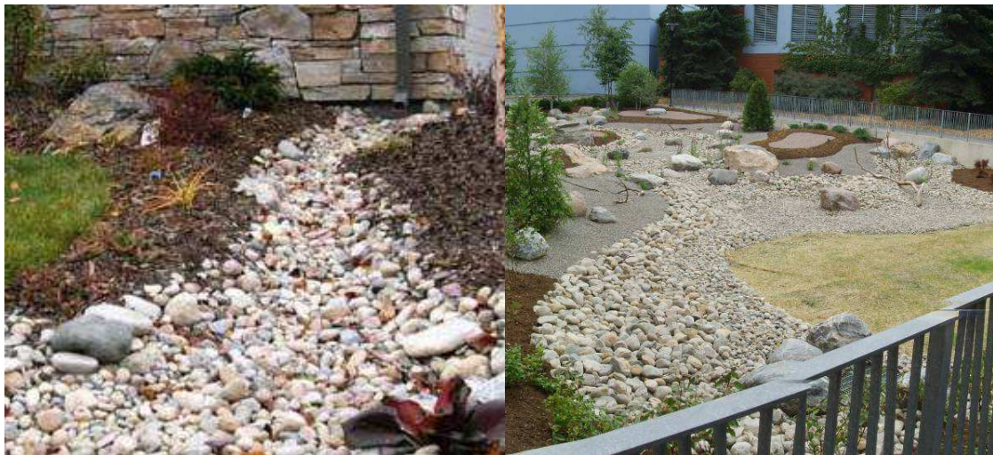
Figure 5. Left: River run stone used to create a dry channel effect for a residential downspout disconnection. (Source: Freeman & Associates, 2008) Right: River run stone used in a xeriscape and bioretention landscape at York University. (Source: York University, 2010)
