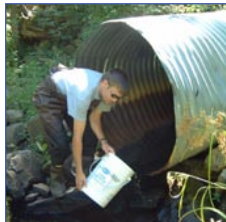
A technician measures the flow of water.
