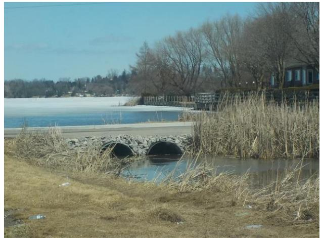
Williams Creek flows through two steel culverts under Old Rail Line before emptying into Lake Scugog.
