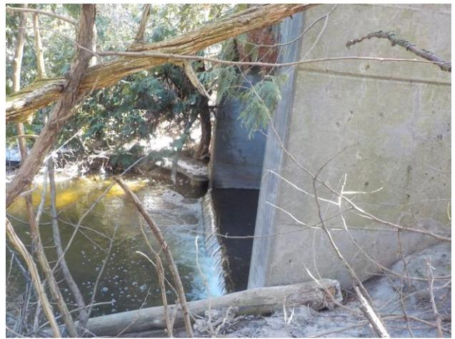
Perched concrete box culvert under Highway 7A (immediately upstream of Station 1).
