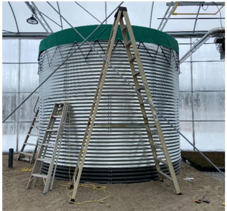
Example of a past approved project for rainwater management. This system catches rainwater that is then used to water plants in a large greenhouse.
